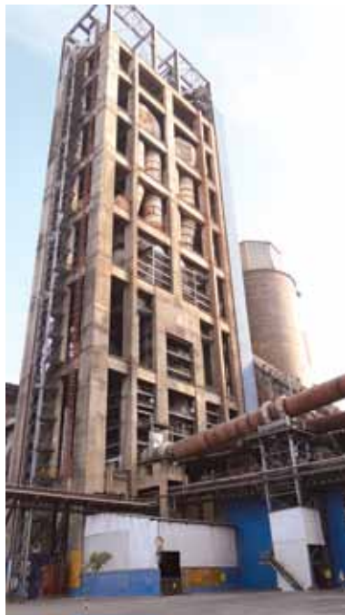
Preheater tower having 6 stages and 2 strings
