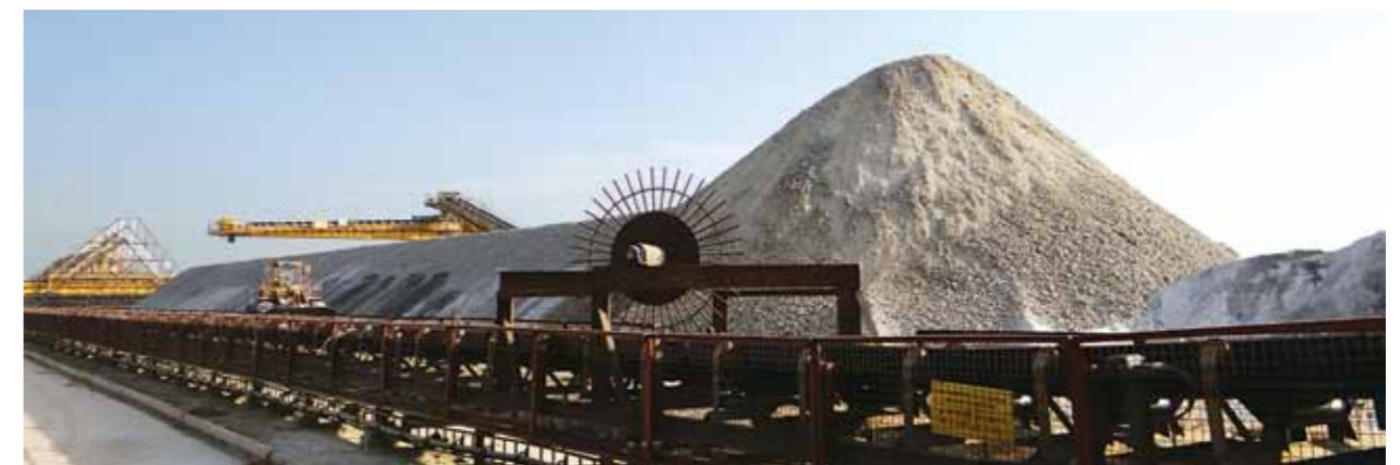
Raw Material Handling section
